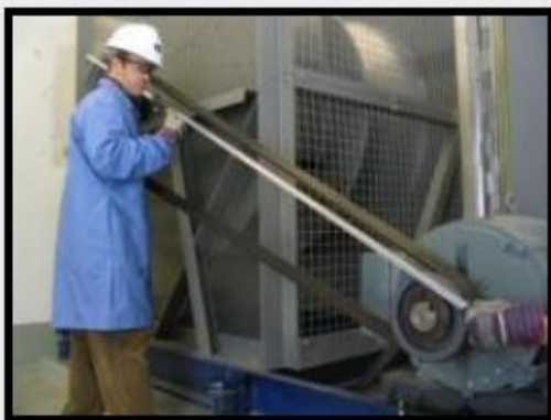
STRAIGHT EDGE – ALIGNMENT CHECK
