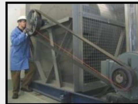
AT1 LASER – ALIGNMENT CHECK
